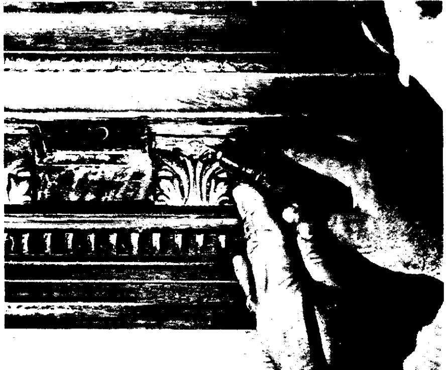
Figure 25. Hyde School, Wood Trim. An elaborately carved cornice had lost detail in a fire. Epoxy patching compound was applied in areas where wood was lost. An electric hand grinding tool was used to restore detail. (Photo: Author)
