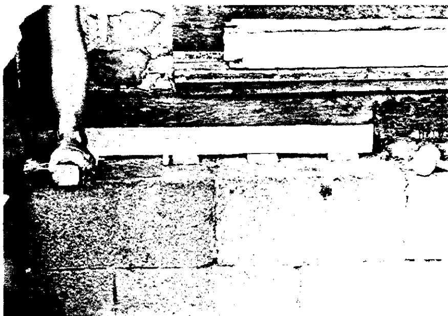
Figure 8. Longfellow House Corner Post and Sill. In the most deteriorated portion of the sill, new wood infill was used. Oak was used to match the material of the original. Wedges front and back were used to tightly position the wood in place. No adhesive was used as the compressive forces really allow no movement of the block once positioned. (Photo: Author)
