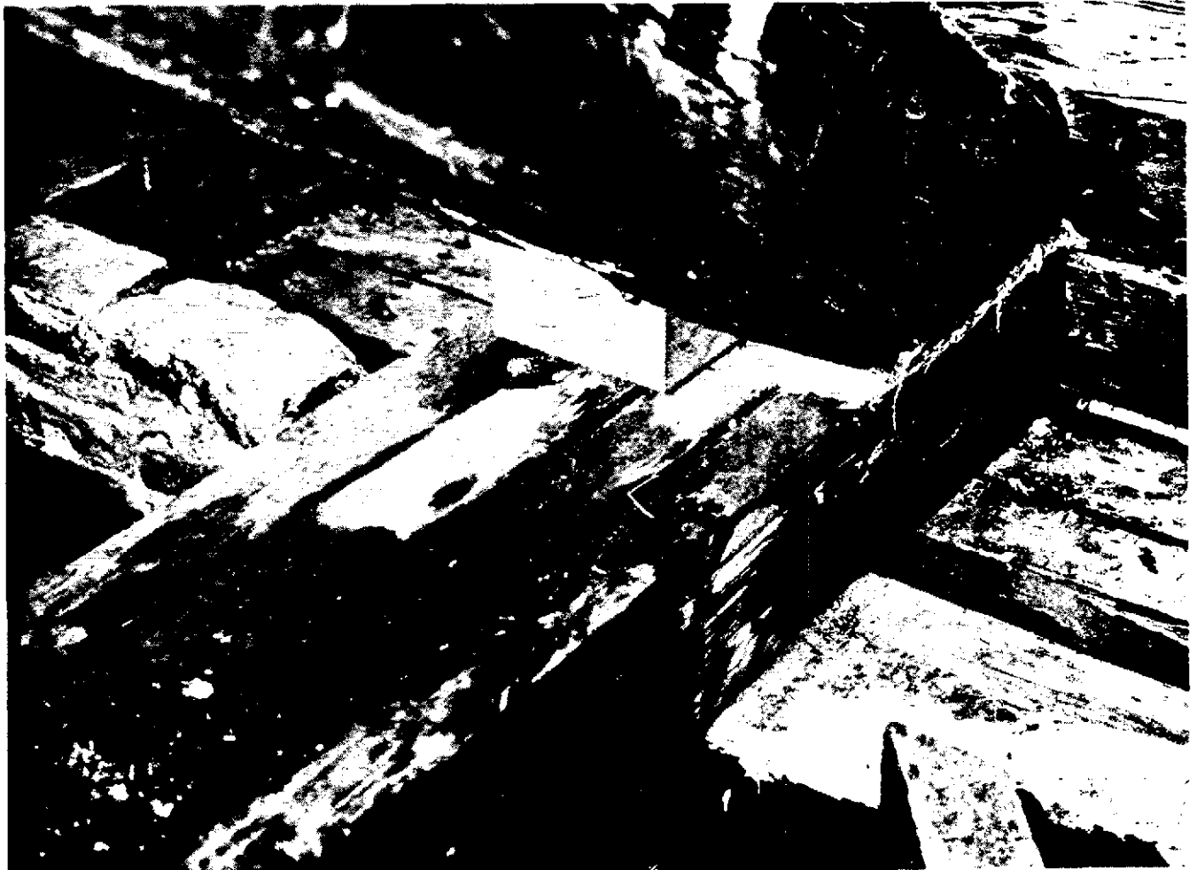
Figure 12. Longfellow House, Central Pediment, Roof Tie Beam. This interior view shows not only tie beam infill, but also the piece used to shim the rafter base. These have been glued in place with epoxy adhesive. It should be noted that the framing elements have lost the mortise and tenon joint that formerly connected them. (Photo: Author)
