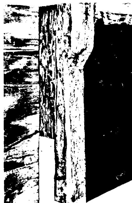
Figure 1. Section of structural oak post consolidated with epoxies. Insect damage had converted this post to a hollow, powdery shell. Wax and clay were used to stop up cracks and holes in the exterior surface while the post was filled with penetrating epoxies. (Photo: Author)
