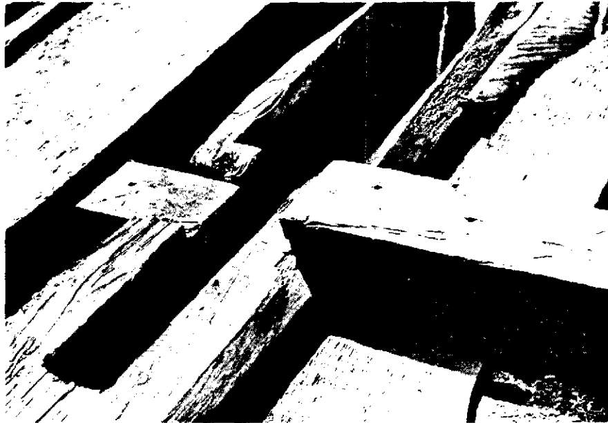
Figure 13. Longfellow House Exposed Rafter Consolidation. View from above after removal of roof slates and sheathing. Deteriorated section of rafter has been removed producing a key-shaped cavity. A purlin is shown framed into the rafter. (Photo: Author)
