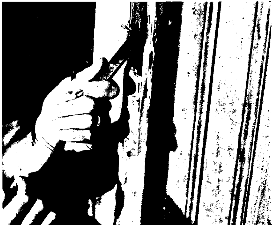
Figure 25. Hyde School, Wood Trim. An elaborately carved cornice had lost detail in a fire. Epoxy patching compound was applied in areas where wood was lost. An electric hand grinding tool was used to restore detail. (Photo: Author)
