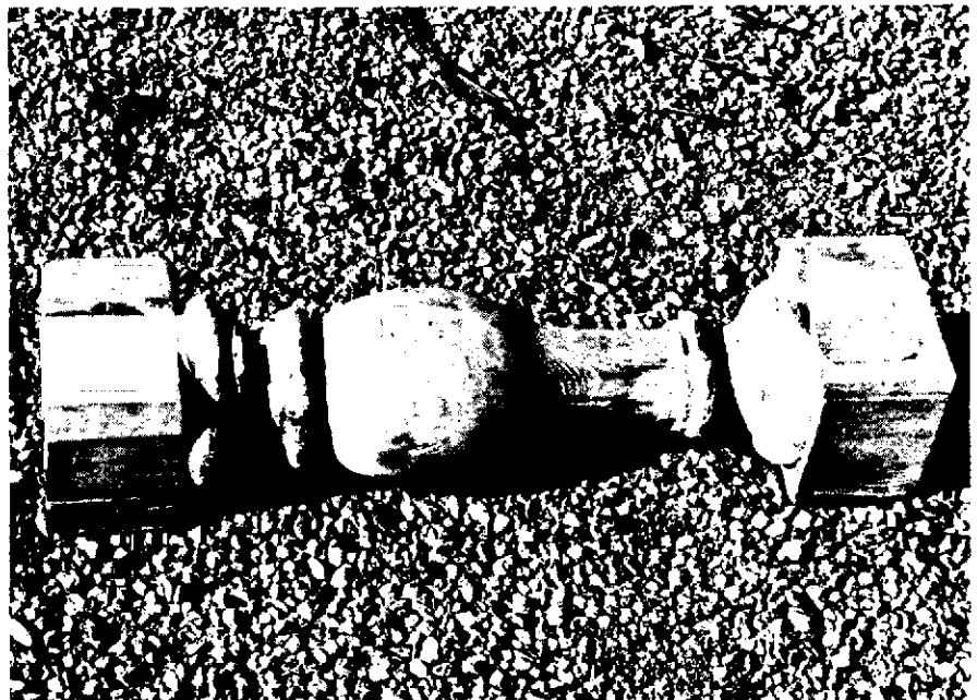
Figure 19. Longfellow House, Turned Baluster. Baluster has been sanded, planed and carved to obtain correct contours. The completed baluster is now ready for repainting. (Photo: Author)
