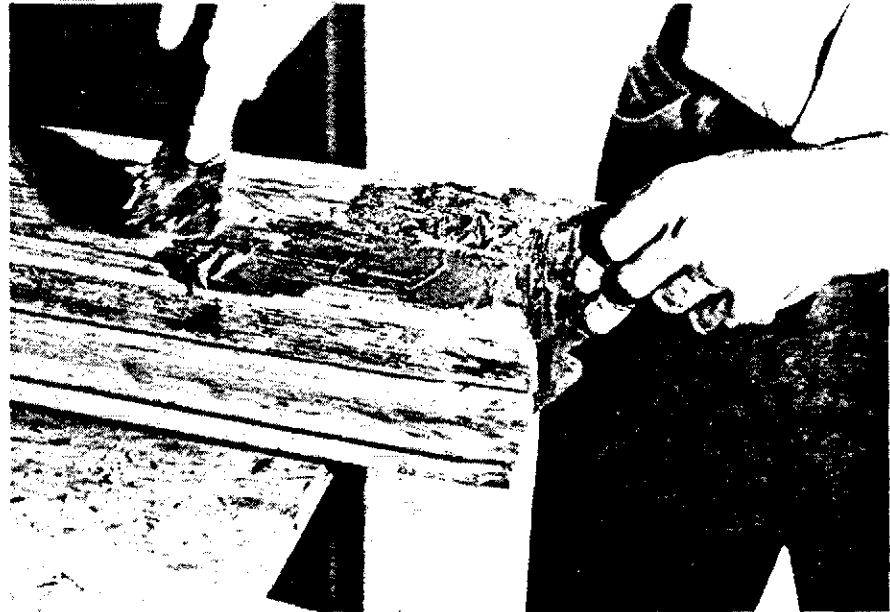
Figure 21. Longfellow House, Porch Handrail. Semi-rigid patching compound No. 1 was used to fill the cracks. A putty knife was employed to force the material into the openings.
