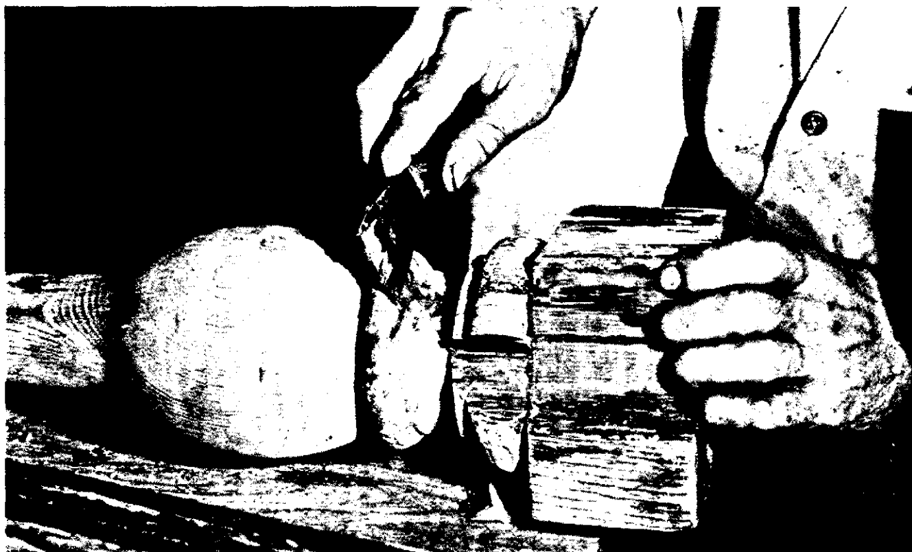
Figure 17. Longfellow House Turned Baluster. Semi-rigid patching compound No. 1 is applied to fill the smaller holes using a putty knife. Care must be taken to prevent air from becoming trapped behind the patch as this will weaken the bond. (Photo: Author)
