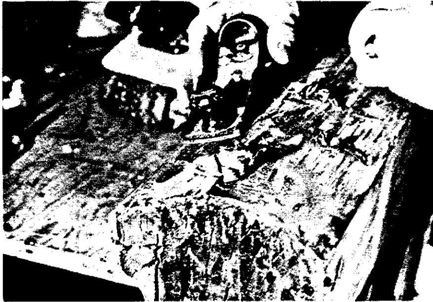
Figure 22. Longfellow House, Porch Hand-rail. The epoxy patching compound is easily planed as well as sanded. (Photo: Author)
