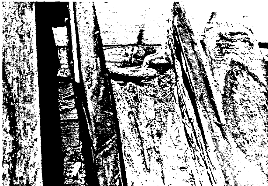
Figure 14. Longfellow House, Exposed Rafter Consolidation. Rafter cavity shown prepared for consolidation by using plywood and caulking to close cavity. (Photo: Author)
